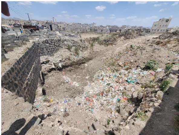
A picture of the culvert from the other side with the backfill that blocks the water from the other side of the road
